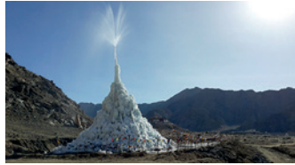
Gravity pressure forces water up through a pipe to form ice stupas that store water for the crop-growing season. ©Sonam Wangchuk
