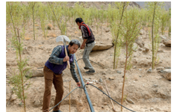
Sonam Wangchuk and a colleague create a drip irrigation network to use water from ice stupas. ©Rolex/Stefan Walter
