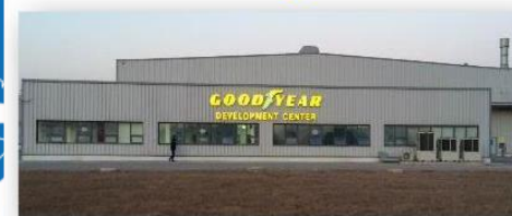
GDC*C in Dalian/Pulandian, China
